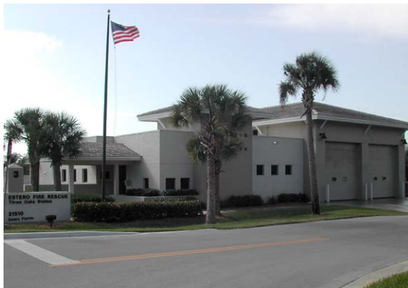
Station 3 – 21510 Three Oaks Parkway
