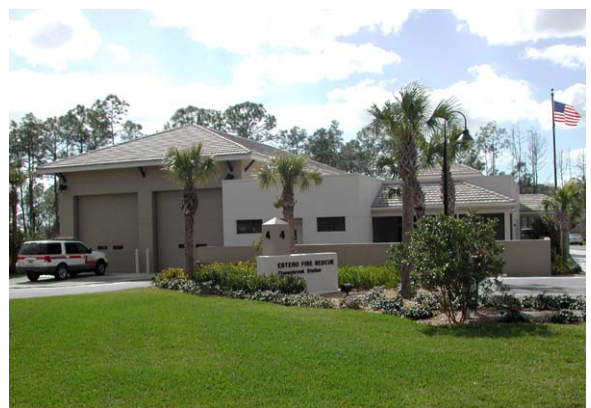
Station 4 – 21300 Firehouse Lane
