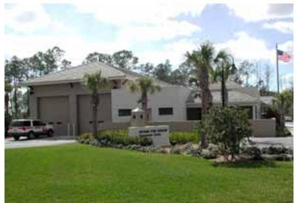
Station 4 – 21300 Firehouse Lane
